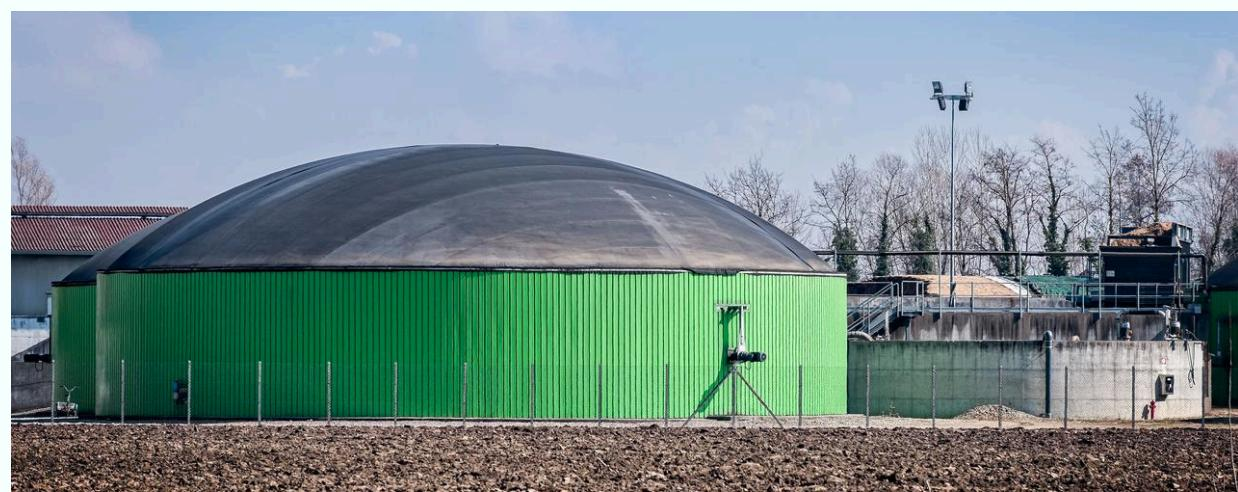
Via project 3229, once manure is stored in the biogas plants, a fermentation process is then used to generate electricity, which is fed into the Dutch national power grid, avoiding further fossil fuel combustion for power within the region.
